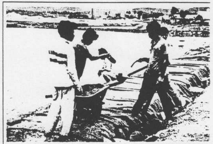
Sand filling operation (Water method)
