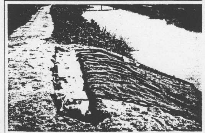
Sand filling operation (Water method)
