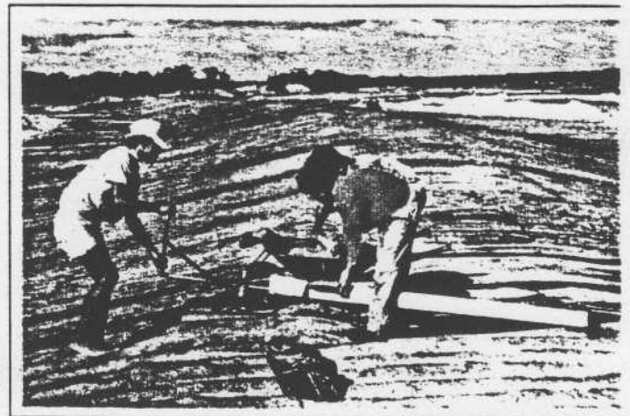
Sand filling operation (Rammer method)
